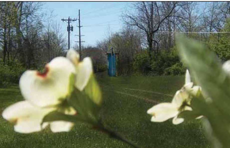
City of Athens production well
